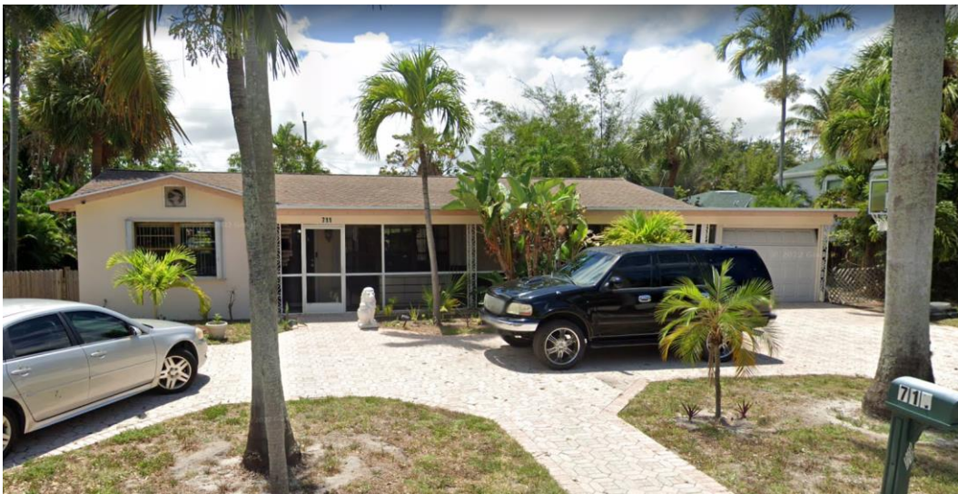
Existing Structure (above)
